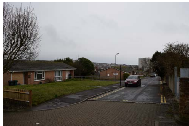
Bungalows 25 and 26 in the foreground, looking south down Ditchling Gardens
