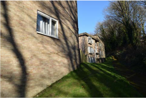
The sloping creates void areas below accommodation.
