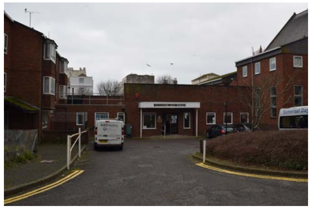
The one storey day care centre with Lavender House to the left
