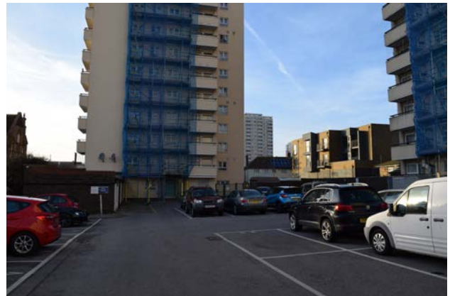
A large area of parking and garages outside Somerset Point
