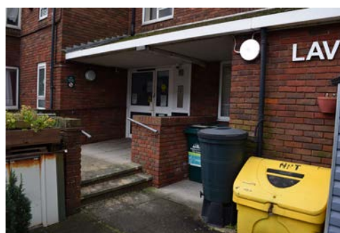
Recycling and salt bins cluttering the entrance to Lavender House
