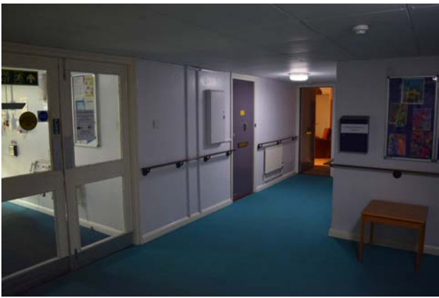
Ground floor flats in close proximity to the main entrance experience noise issues
