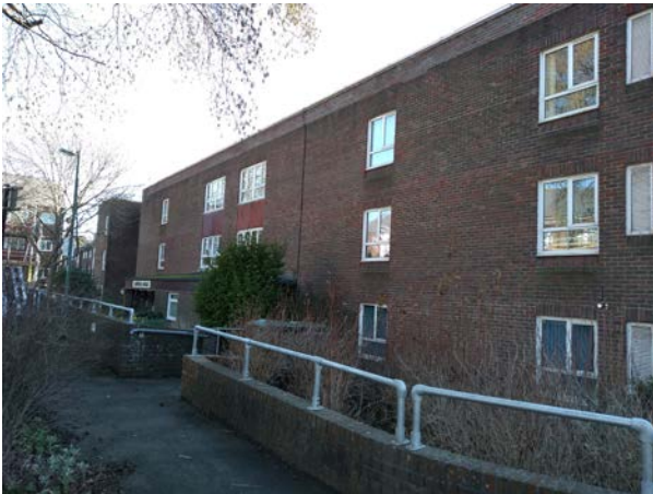
The entrance faces north and the front door is down a ramp however it is well sign-posted
