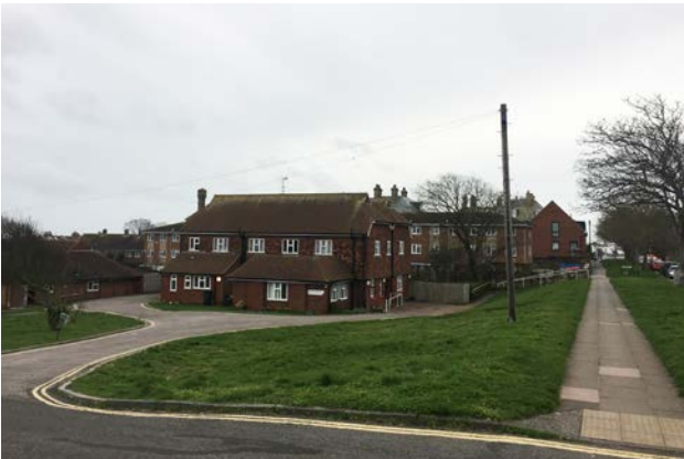
The nineteenth century farm house converted into flats and communal facilities.
