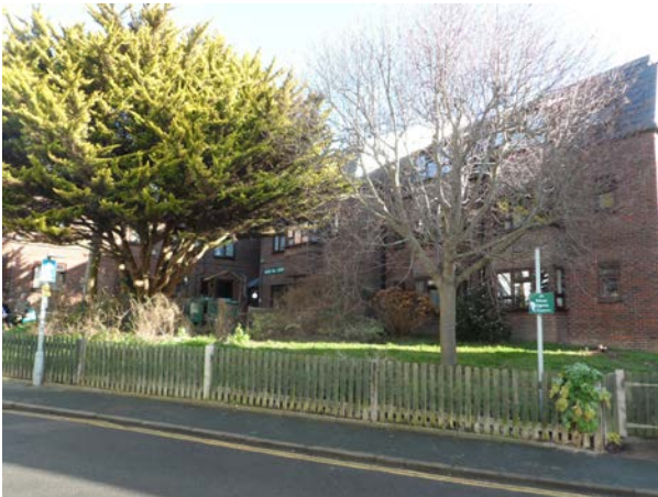
The front garden and entrance. Set back from the building line of Kingsbury Road, it isn't obvious at first, but the main entrance is apparent once you are on site.
